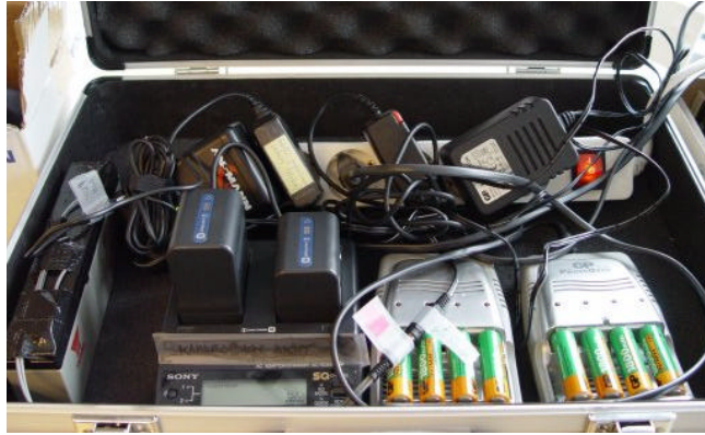
Figure 6. One set of the batteries was being charged while the other set was in use
